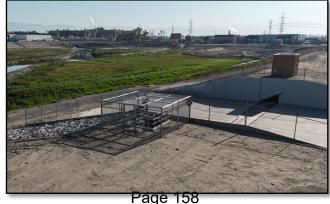
Outlet Control Gate/Rubber Dam System
